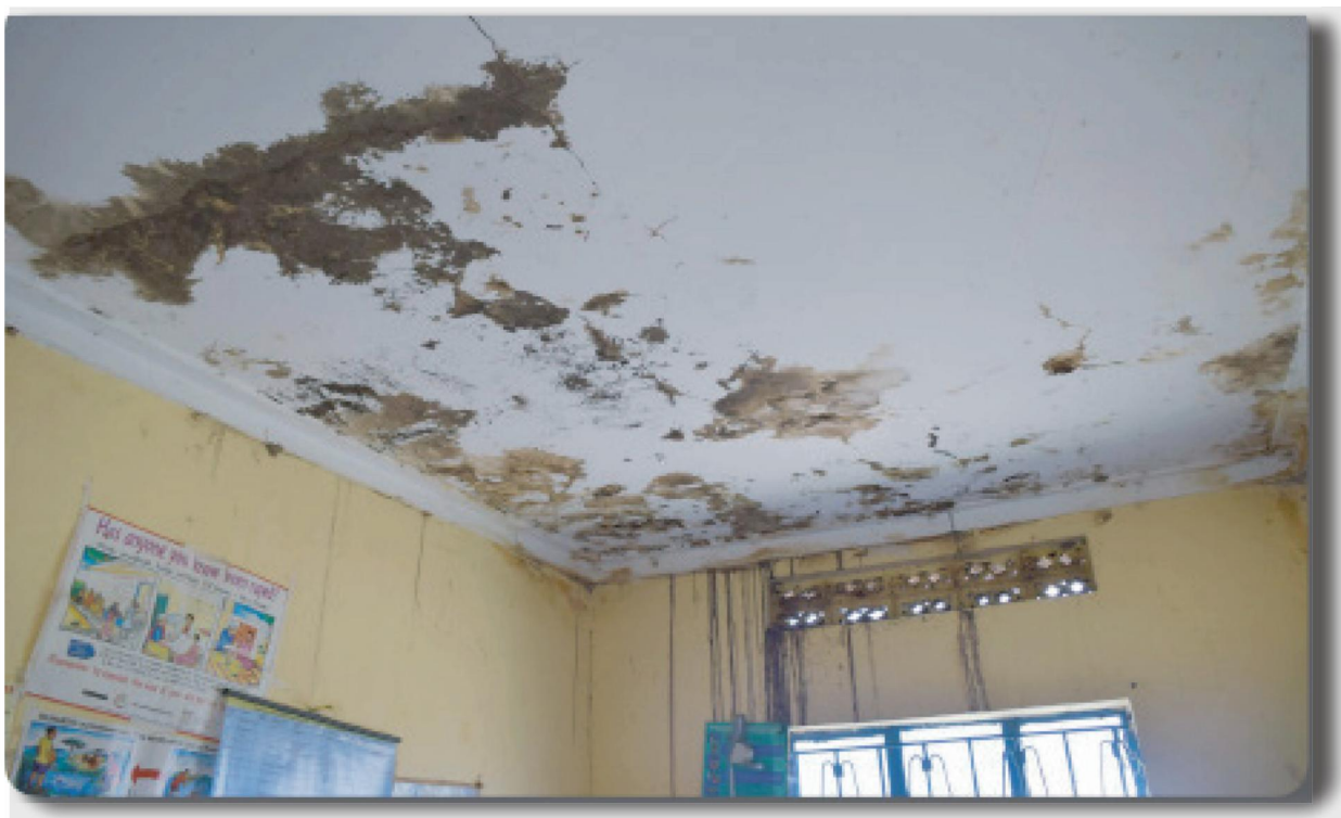
Portion of the ceiling of the Health Centre which has been infested by bats.
