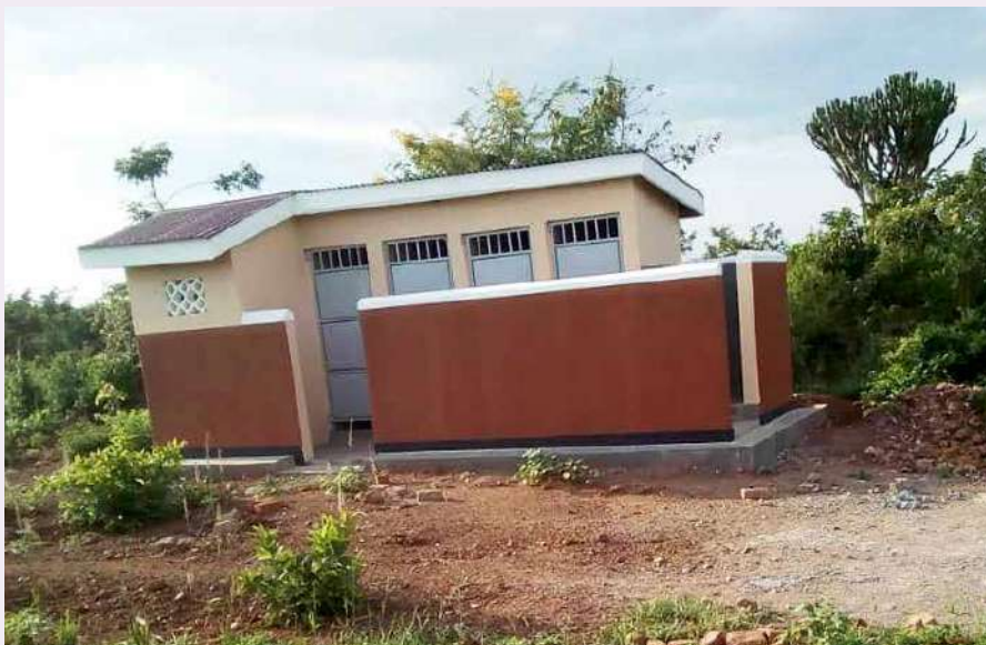
A four stance pit latrine recently constructed at Nakitokolo Primary School
