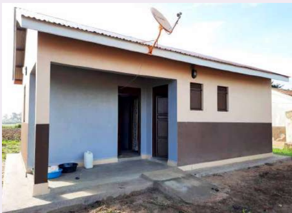
Staff quarter constructed at Mukongoro Health Centre III, Kumi District to accommodate the facility in-charge officer
