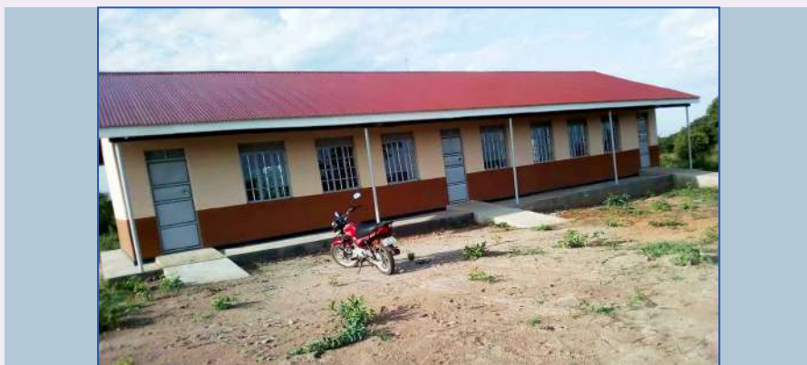
A two classroom block constructed at Nakitokolo Primary School following the EOC ruling
