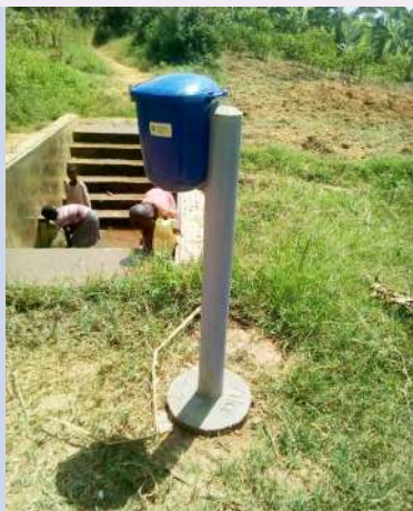
A chlorine tank constructed at Bukewa East village water point.
