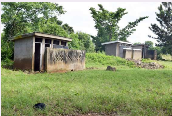
The old latrine structures (on the left) and the new latrine structure (on the far right) at Bukewa Primary School
