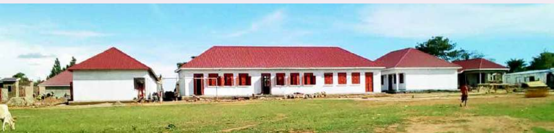
Some of the newly constructed structures with classroom blocks, staff houses, administration office and latrines at Bukewa Primary School
